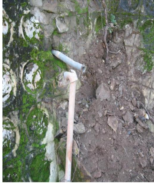
**View of Cracked Pushta and Broken Intake Pipeline at Dhaur Barsudi WSS**
